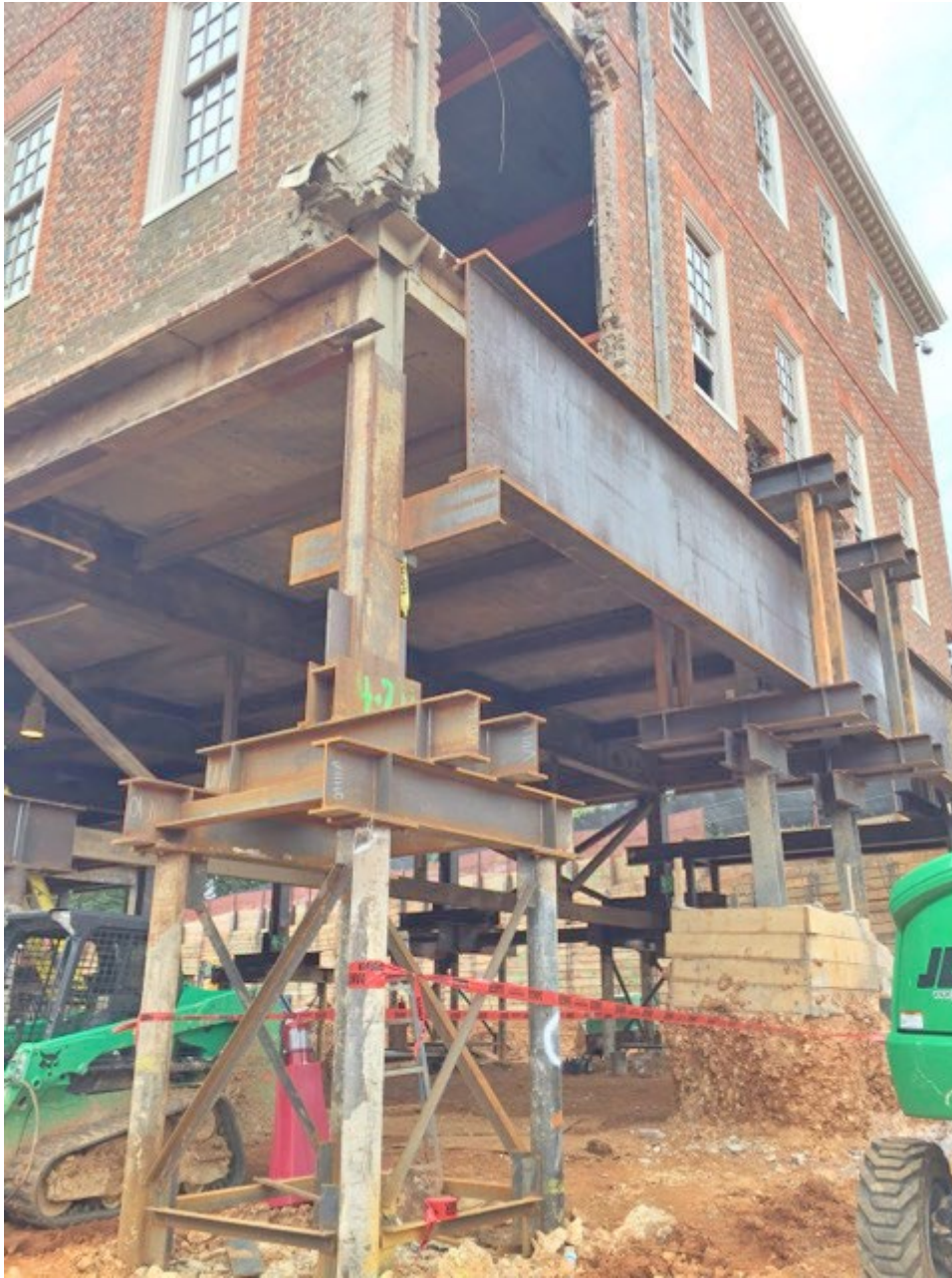
Picture 2. Three existing columns were transferred prior to being removed.
