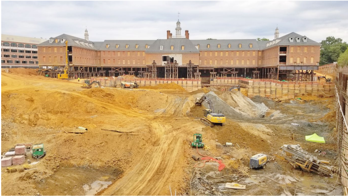
Picture 3. The entire “H” shaped historic building was lowered 7 to 12 feet
