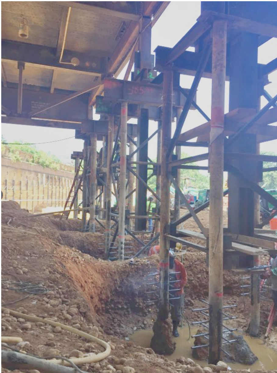
Picture 1. Existing foundations were removed with columns were extended 12 foot.
