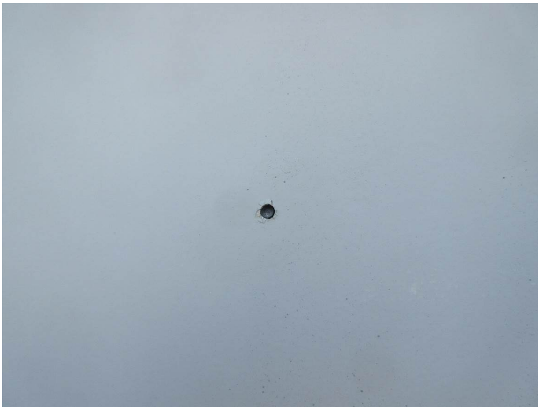
Typical overdriven fastener
