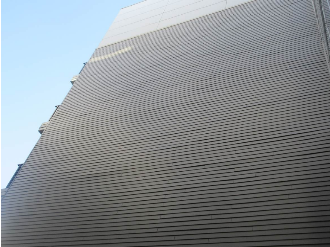
Waviness of fiber cement lap siding
