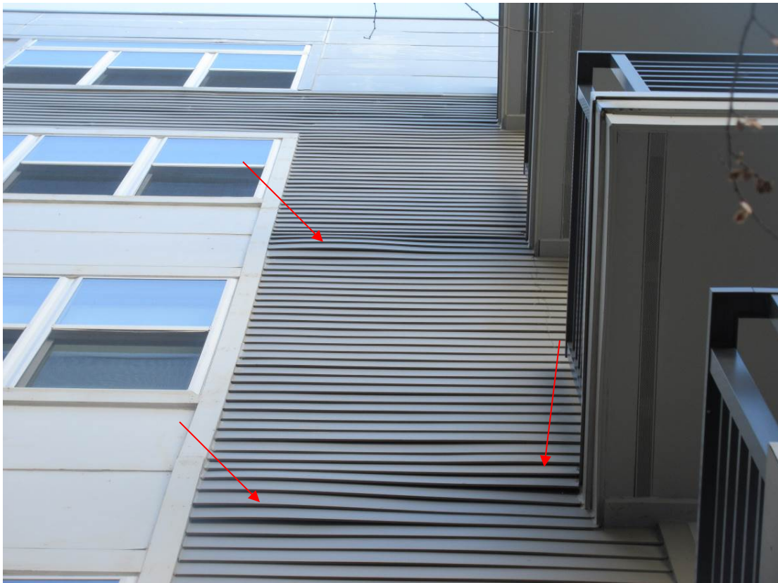
Significant bulging of fiber cement lap siding
