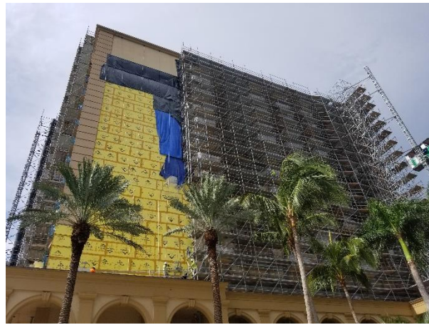
New wall sheathing placed after removal of stucco.
