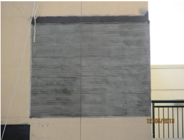
Scratch coat applied at a stucco repair area.
