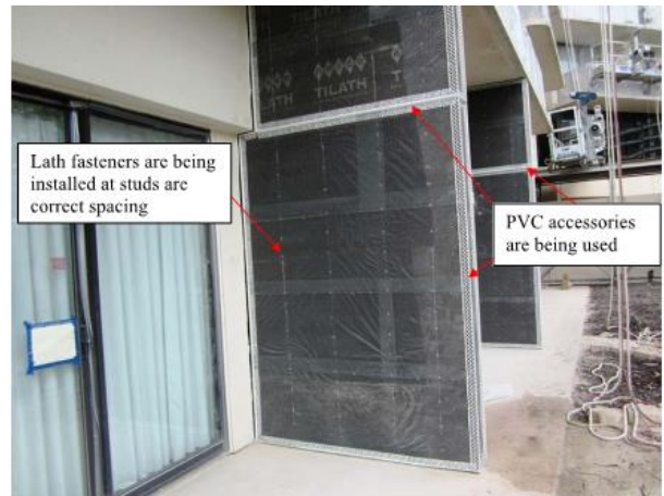
New lath and PVC accessories installed.
