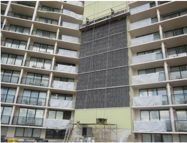
New lath and PVC accessories installed over new weather resistive barrier.
