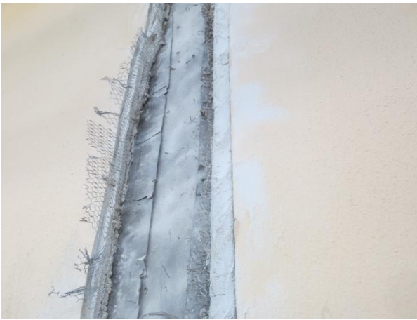
Deteriorated stucco removed from façade.
