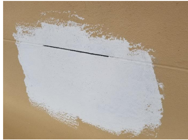
Application of primer on repaired stucco wall.
