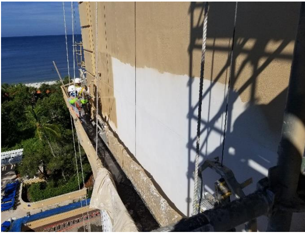
Application of primer and coating on repaired stucco wall.
