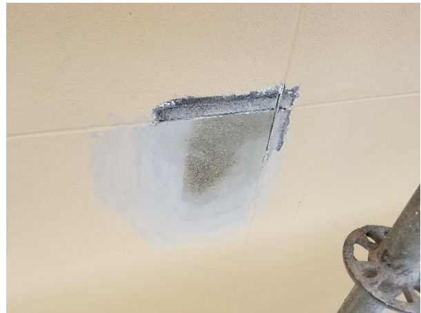
Stucco patch finished to match that of existing stucco.
