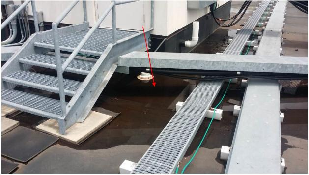
**Photo 3** – Ponding water at roof
