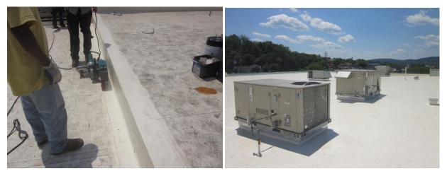
**Photo 4** – Heat welding seams in new roof
