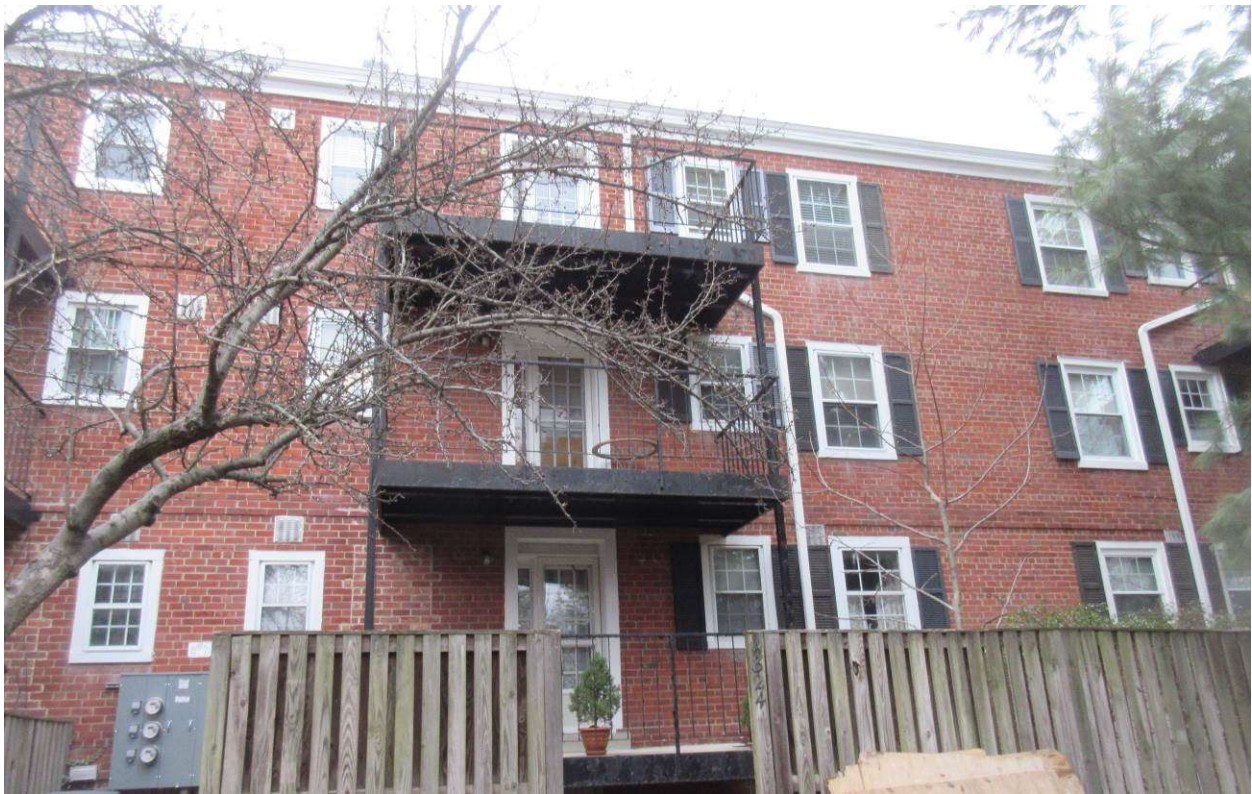
Overall view of steel framed balconies
